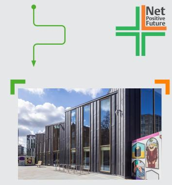
BAM recently completed the King's Cross Sports Hall, it is constructed out of 838m<sup>2</sup> of timber (690m<sup>3</sup> of CLT and 147m<sup>3</sup> glulam, from 100% PEFC chain of custody sources). But it is more than just a leisure facility – it has been designed to have multiple uses and is highly adaptable for a long lifespan.
