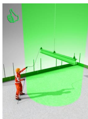
Fig 3 – Correct use of tag line
