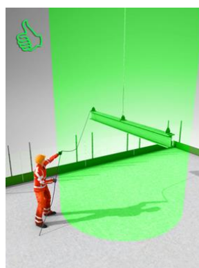
Fig 3 – Correct use of tag line
