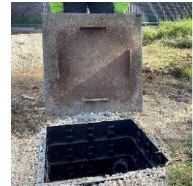
Cold rolled asphalt infill, footpath covers and tanged plates for pedestrian routes
