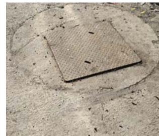
Cold rolled asphalt infill, footpath covers and tanged plates for pedestrian routes
