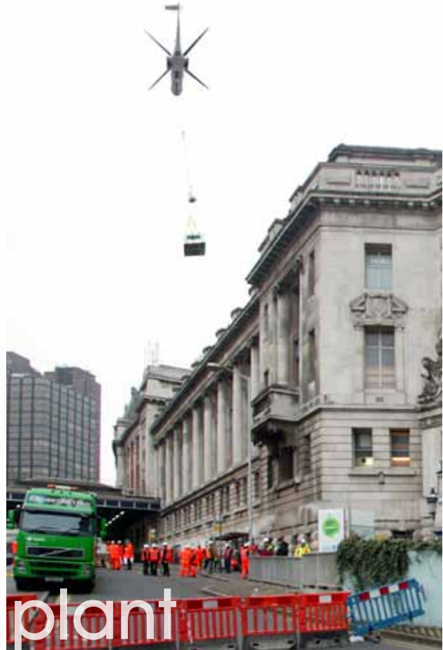
Plant lift onto Waterloo Station roof via helicopter for Network Rail
