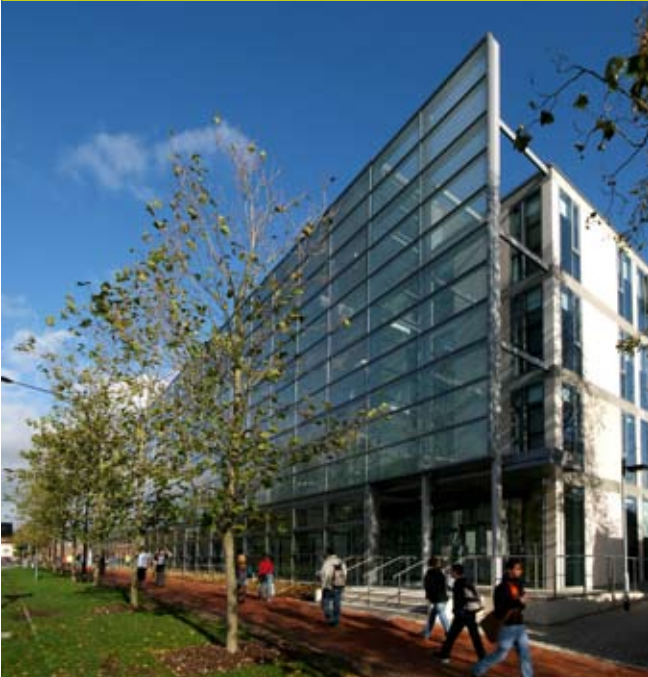
EEE Building, Southampton University
