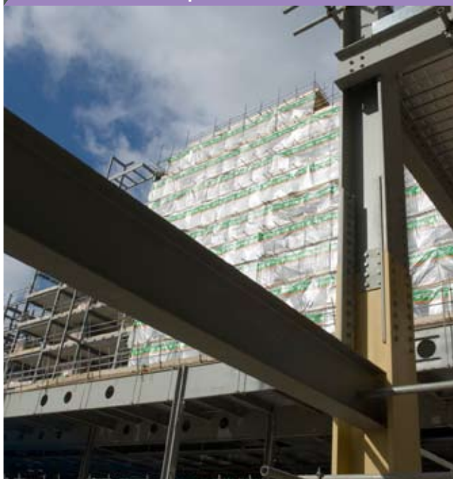
Progress at the Sainsbury's mixed development project, Milton Keynes
